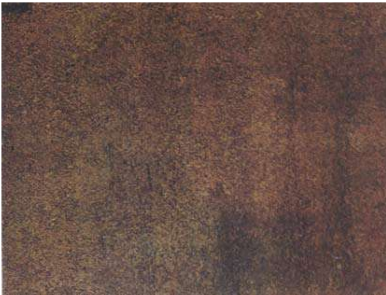
Scraping and wire-brushing
