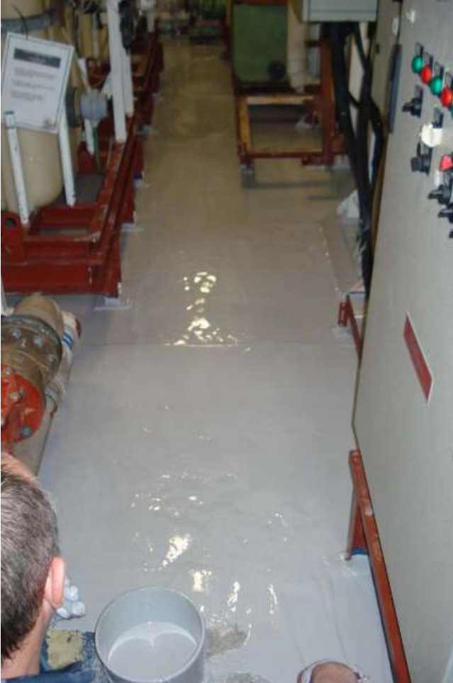
Note: Thick section applied in 1 coat
