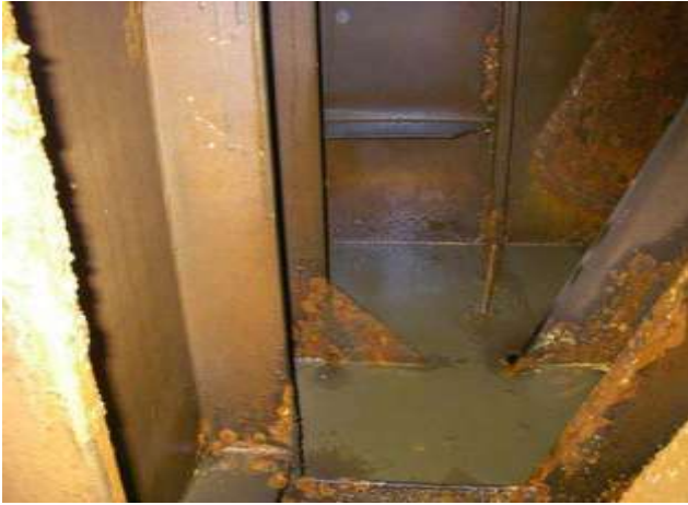
Black slime deposit at surface can indicate MIC
