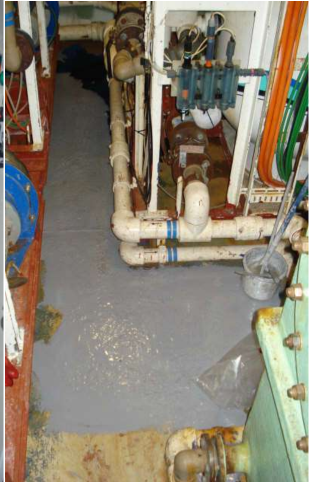
Note: Existing paint system
