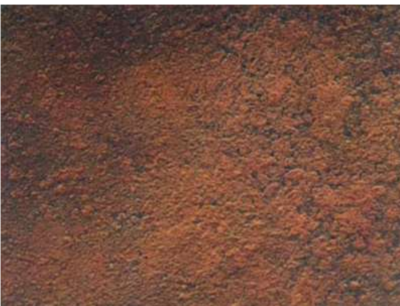
Scraping and wire- brushing
