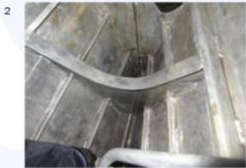
Photographs • Nos. 1 & 2 Surfer boats 2612 & 2601 before surface preparation, respectively • Nos. 3 & 4 Surfer boats 2612 & 2601 after surface preparation, respectively • Nos. 5 & 6 Surfer boat 2612 after application of Chemco system • Nos. 7 & 8 Surfer boat 2601 after application of Chemco system
