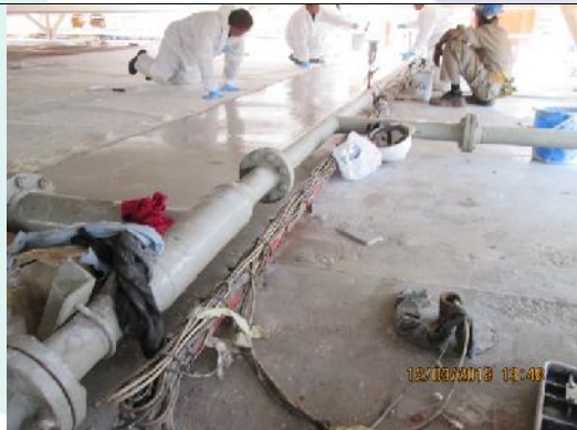
Pic 20: Laminating in action, shipyard assistance present.
