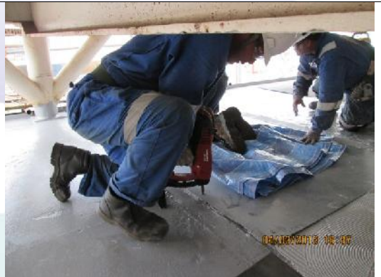
Pic 15: Gunning the first plate down using the Hilti Compressed Air Gun model GX120.
