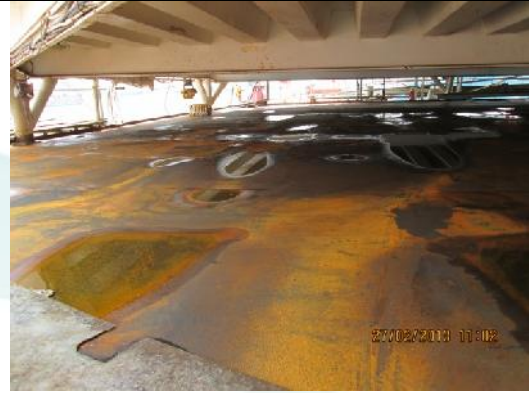
Pic 6: After wash surface ready to prime with Chemco RS 500P
