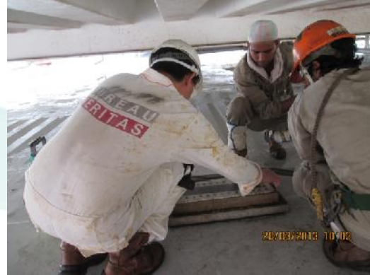
Pic 24: Vacuum Test in action with BV inspector present...passed the test!
