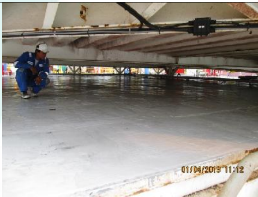
Pic 25: Finished Work Completed after testing ready for service
