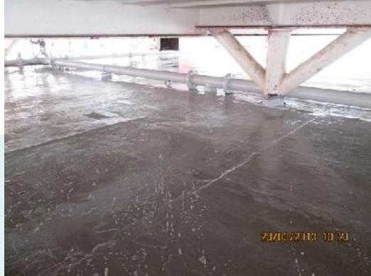
Pic 23 Completed work after top coat just prior to Vacuum test
