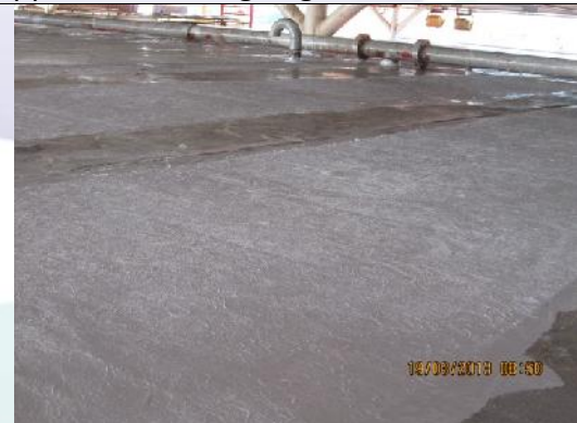
Pic 21: Completed surface ready for next process.
