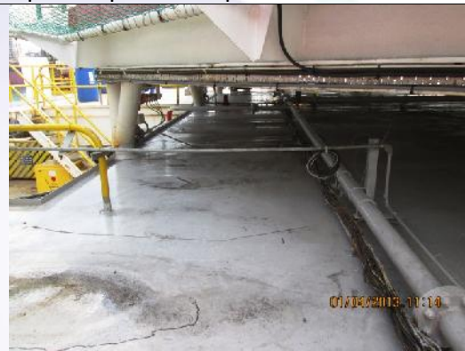
Pic 26: Finished Work Completed after testing ready for service.
