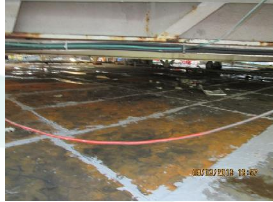
Pic 17: Plates laid over wide area not the glue line between plates ensuring full bonding even on the edge.
