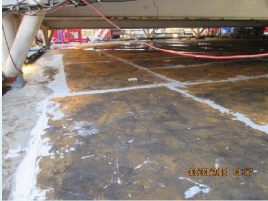
Pic 16: Plates laid to over 80% of the surface area.
