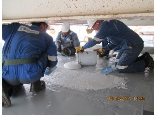
Pic 12: First step in preparation for the plate apply a bed of wet material suitably prepared, the men call this "mud"
