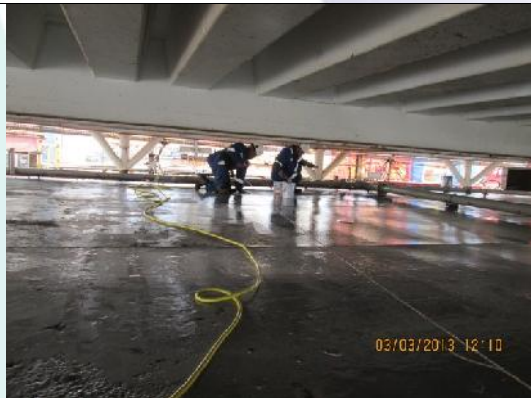
Pic 9: Priming of surface in progress.
