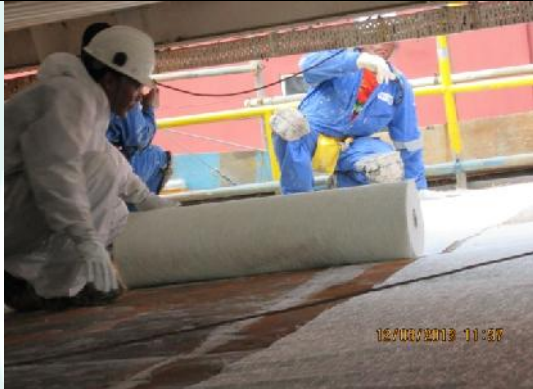
Pic 18: The First Laminating Cloth laid out
