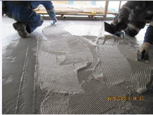
Pic 14: The entire surface has the mud applied, the plate is applied whilst the mud is still wet forming 100% glue line
