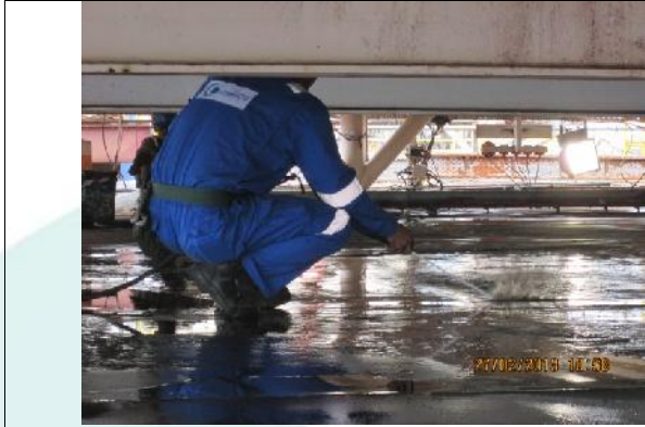
Pic 5: Washing the deck after the Power wire brushing was complete
