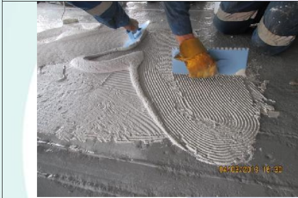
Pic 13: Notched trowel used to spread the mud evenly.
